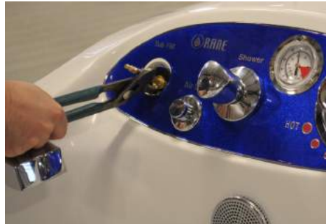
Step 8: Use tongue & groove pliers on base of valve stem and remove.
