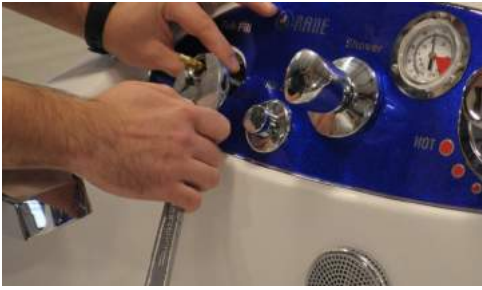
Step 5: Using a crescent wrench, remove part C (fig.1).
