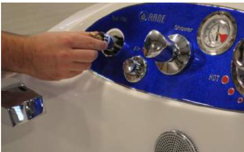
Step 13: Using a crescent wrench, Re-install part C (fig.1)/
