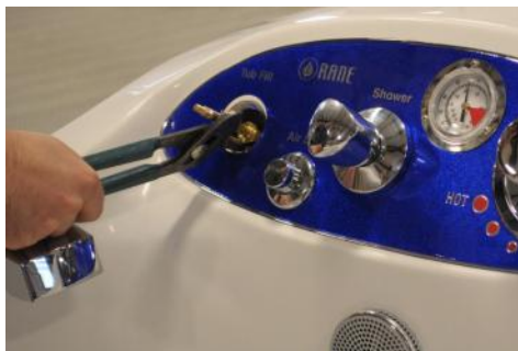
Step 10: Use tongue & groove pliers on base of valve stem and tighten until it stops. Be careful not to over tighten and snap the stem.
