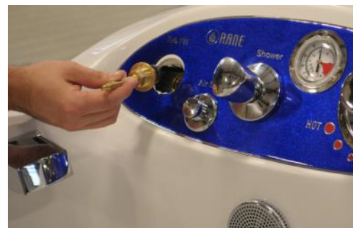
Step 9: Insert and carefully thread in new valve stem. Hand tighten.
