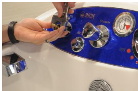
Step 13: Using a crescent wrench, Re-install part C (fig.1)/
