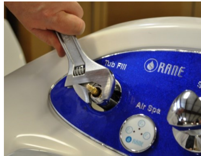
Step 11: Re-install part E (fig. 1). Note: Do not over tighten.
