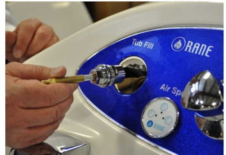
Step 9: Insert and carefully thread in new valve stem. Hand tighten.
