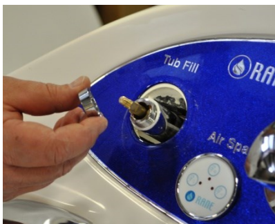
Step 13: Using a crescent wrench, Re-install part C (fig. 1).
