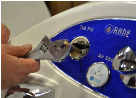
Step 10: Use crescent wrench on square tip of the valve stem and tighten till it stops. Note: Be careful not to over tighten and snap the stem.
