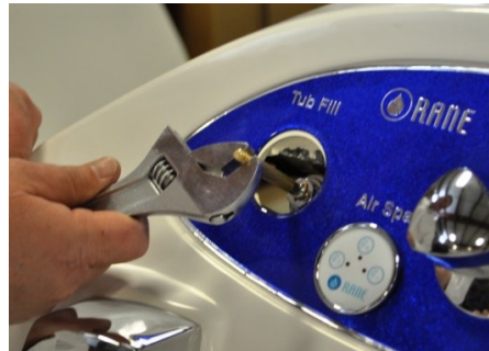
Step 8: Use crescent wrench on square tip of the valve stem and remove.
